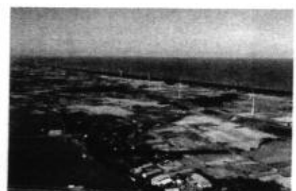
Large-scale wind farm (13,500-kW)
