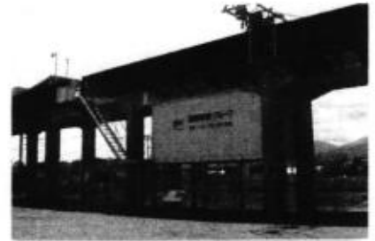
Electrical control room and grid connection point
